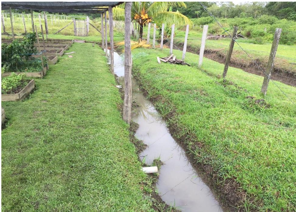
Figure 66: Flood trenches constructed at *Green Leaves* to manage floodwaters
